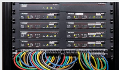
Network gateway bristling with LAN cables (VHF on left, UHF on right)
